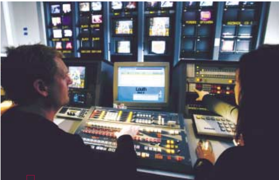
FOX Digital, the network's broadcast center for the United States in Los Angeles, is equipped with an array of Grass Valley products.
